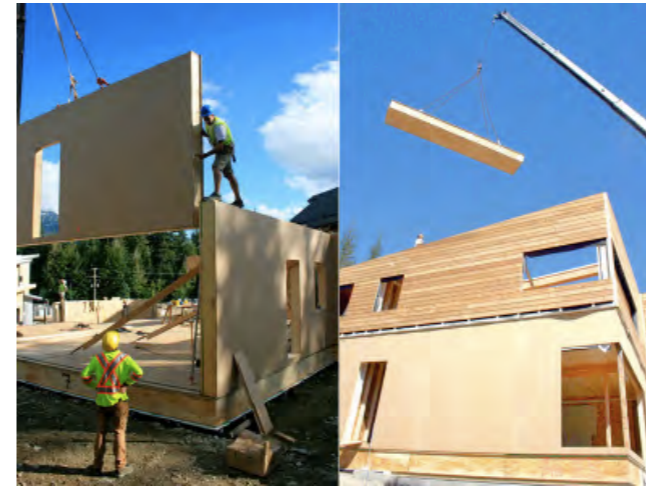
Prefabricated panels being delivered to site
